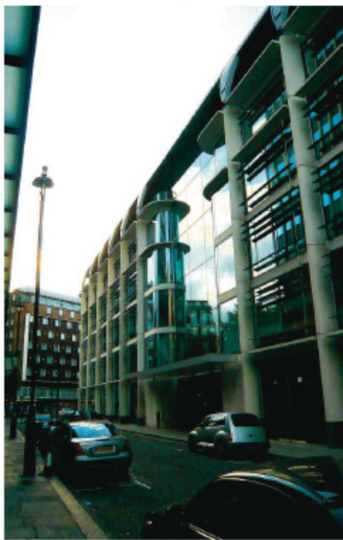
At Shaftesbury Avenue in London, Welcome Gate was brought in to review the physical safety, and it chose products from Gunnebo.
